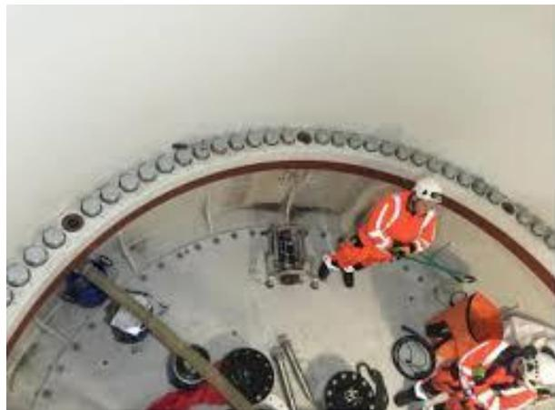
In order to monitor the health of these connections, regular inspection is needed, requiring costly vessel time and / or maintenance procedures.
