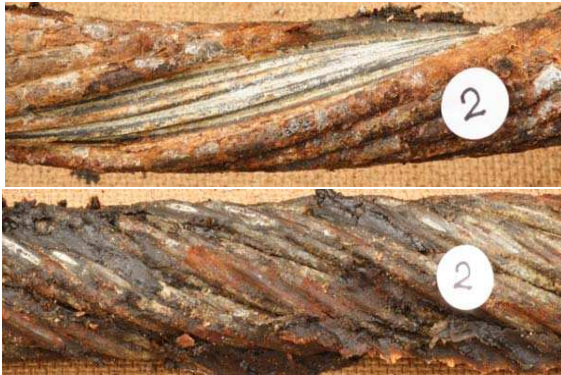
Outer strand (above) and IWRC (below) from 6-strand upper segment of mooring rope with A-gal outer wires, after 13 years deployment in North Sea.
